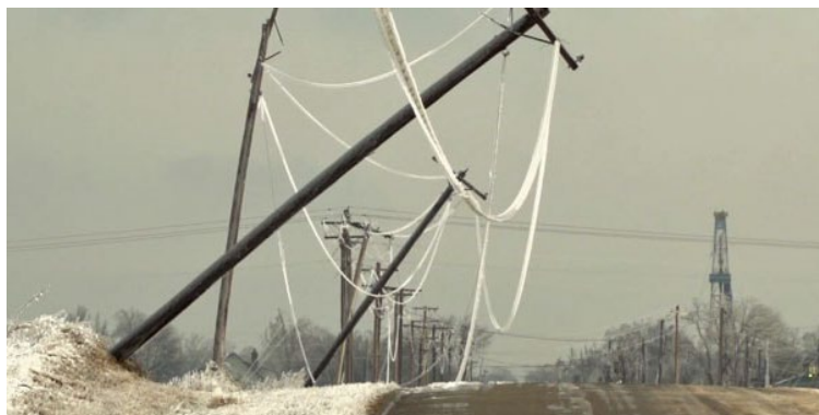
Figure 1 – Damaged power line
